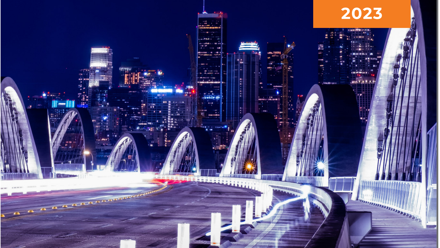
Sixth Street Bridge | Los Angeles
